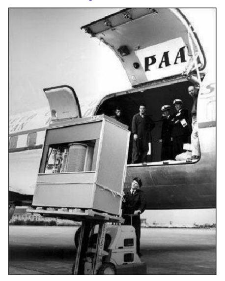
Date: 26th of September 1956 4.4 MB (Megabyte) Hard Disk Weight aprox. 1ton
